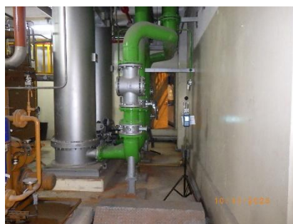
Stream Turbine Lube Oil Skid (Block 2)
